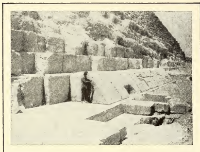
FIG. 75.—THE FACING SLABS STILL INTACT OF THE GREAT PYRAMID. ( Phot. Covington. )
