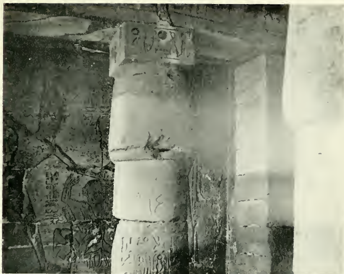
The Temple of Wady Abâd. The east end of the Portico. The square pillar was built in Græco-Roman times to support the broken architrave.—Page 155.
