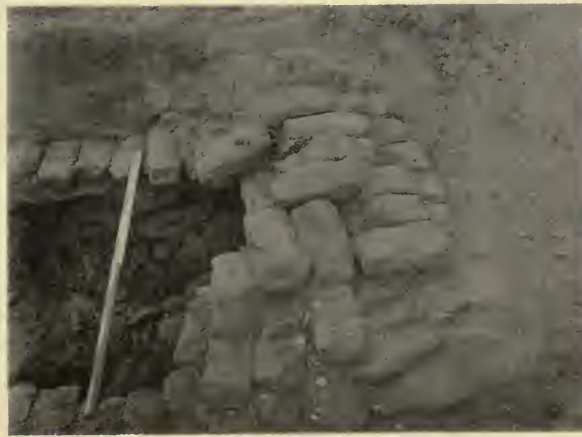
f. Construction of vault at northeast corner.
